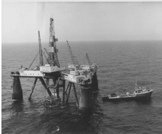
Rig Sea Gem UKCS 1965 Legs collapsed- 13 dead
