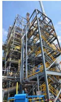
Small Pilot (100kW th -3MW th )
