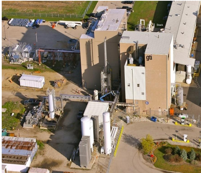
5 MW th fully integrated and instrumented test bed for gasification, gas processing, and syngas synthesis technologies.
