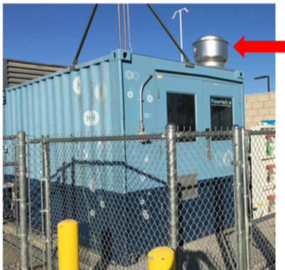
Compressor enclosure with mechanical ventilation (red arrow shows exhaust outlet)
