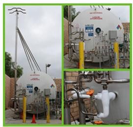
Another unique challenge presented by liquid hydrogens cryogenic temperatures is condensation. Specifically, condensed air, which can form on uninsulated LH2 equipment and present a hazardous situation as oxygen enrichment creates explosive conditions near the liquid hydrogen system.
