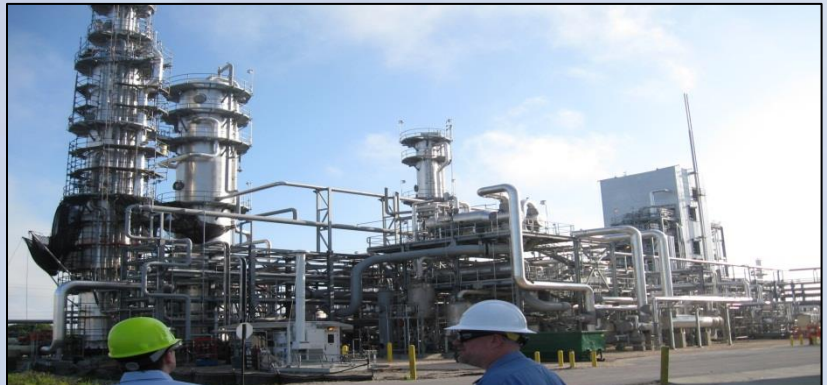
Completed Construction – 50-MWe Demonstration Project
