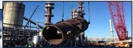
Installing WGS Reactors
