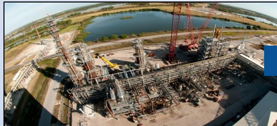
Installing Carbon Capture System
