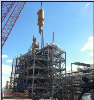
Installing Warm Syngas Desulfurization Equipment
