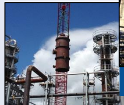
Installing WGS Reactors
