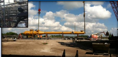
Installing Warm Syngas Desulfurization Equipment
