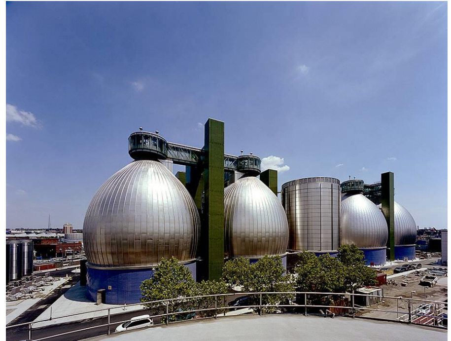
Picture of Newtown Creek wastewater treatment plant in Brooklyn, NY.
