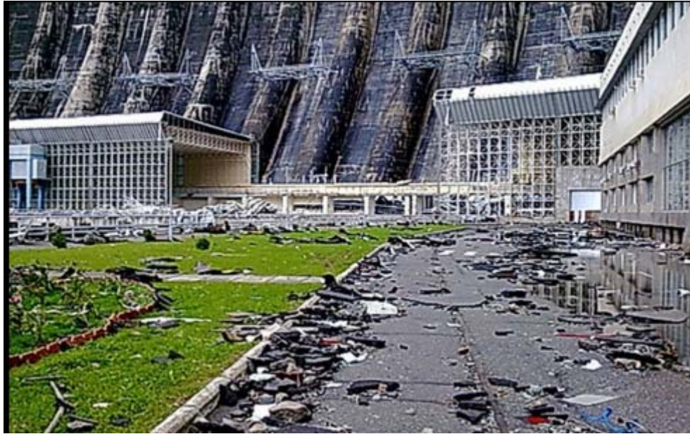
Figure 5.6 The power station after the accident, with the roof of the turbine hall partially collapsed
