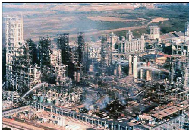
Explosion and Fire Pasadena, Texas October 23, 1989
