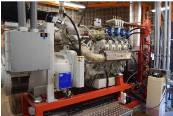
375kW CHP Engine/Generator Set Source: DGSD
