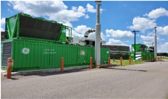
CHP Units 1 and 2 – Total 1.26 MW Biogas Fueled Source: St. Cloud NEW Recovery Facility
