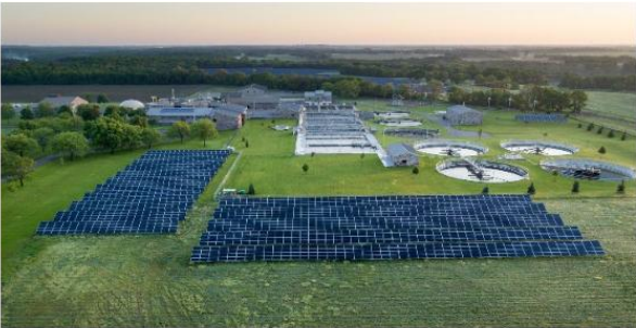
220 kW (left, installed 2017) and 240 kW (right, installed 2020) Solar Arrays Source: St. Cloud NEW Recovery Facility
