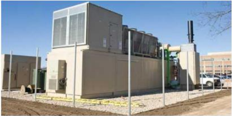
CHP Engine Generator Set with Heat Recovery and Gas Clean Up Source: DOE CHP TAP
