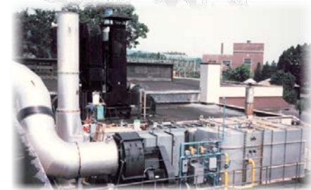
20,000 CFM TO Textile Manufacturing Facility
