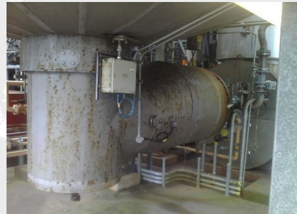
System Burner (Start-up Only)
