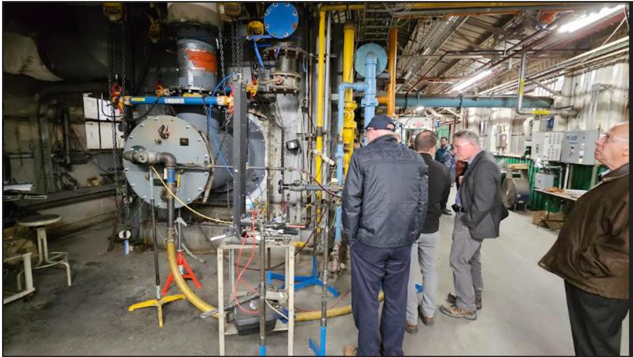
Burner on exterior of Metals Heat-Treating Furnace
