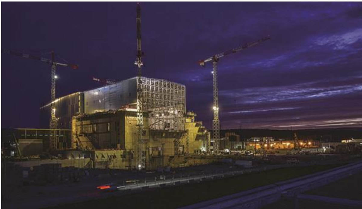
1. The ITER project, shown during construction in February 2020, will be the first experiment to create a “burning,” or self-sustaining, fusion plasma. This photo shows
