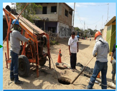
Cleaning (Dredging) of Sewer Lines/Pipes
