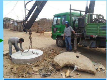
Repair/Replacement of Dilapidated Manholes
