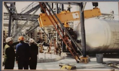
INSTALLATION OF THE 147 TONNEUR TANK AT THE BAYVIEW SITE © 1997 OGP
