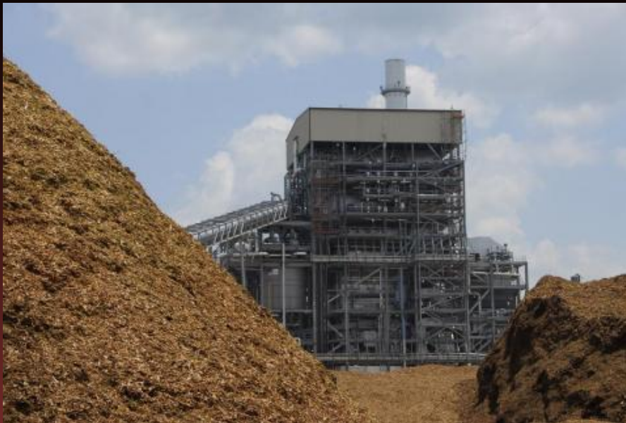
Ground view of Operating Biomass Gasifier
