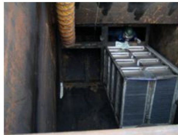
Retrofitting an Existing CPI unit--Photo 1
