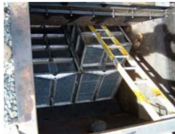
Retrofitting an Existing CPI unit--Photo 2
