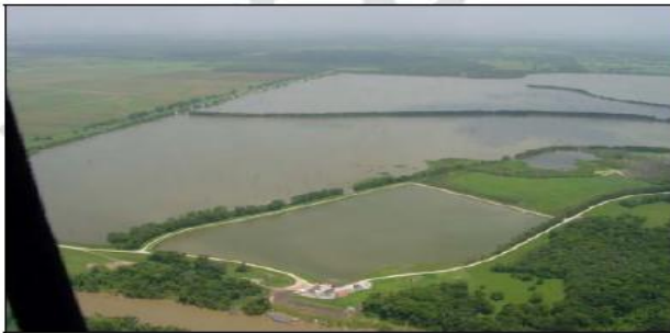
Figure 1-3. Harris Reservoir with Pre-sedimentation Basin and Brazos River Intake and Pump Station in Foreground
