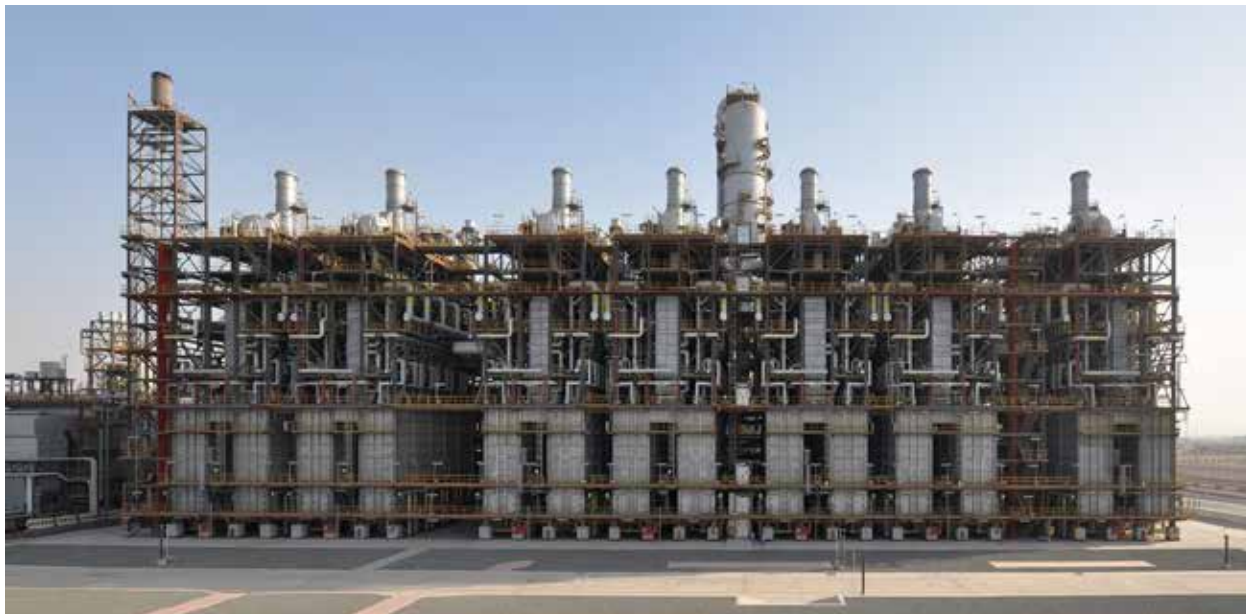
▲ Figure 5. At the heart of the ethylene production process are the steam-cracking furnaces. Here, seven cracking furnaces are shown at the Borouge 2 Ethylene Plant in the United Arab Emirates. Photo courtesy of Linde Engineering.
