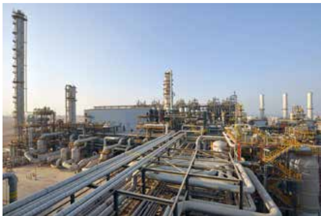
▲ Figure 6. The recovery section of the ethylene production process separates and purifies the products from the cracked gas stream. Recovery involves cryogenic separation of the gas in a series of distillation columns — ultimately producing high-purity ethylene. Shown here is the recovery section of the Borouge 2 Ethylene Plant in the United Arab Emirates. Photo courtesy of Linde Engineering.
