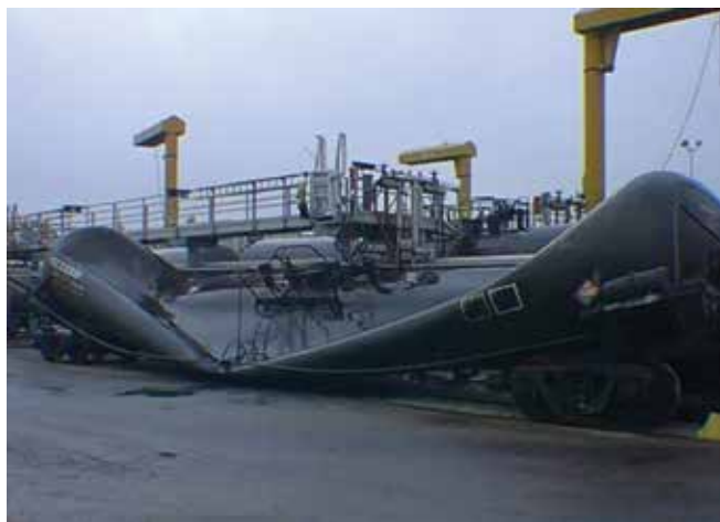
▲ A railcar collapsed after a steam-out process because it was not properly vented.
