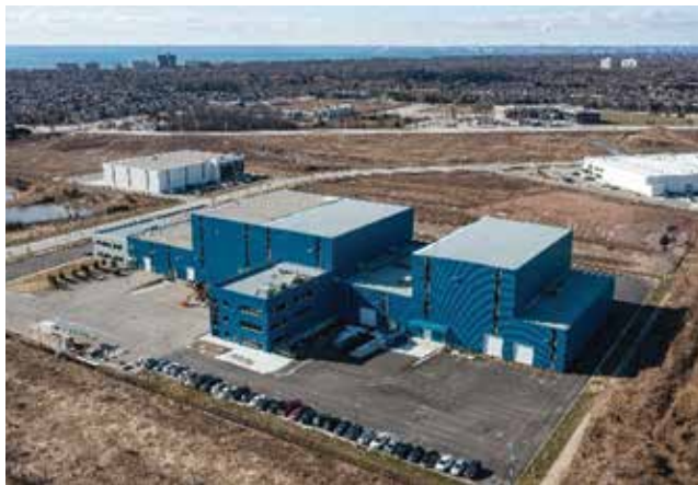
▲ Figure 7. Large vertical windows were incorporated into Zeton's building design to introduce more ambient light. Increasing passive lighting reduces energy consumption and improves working spaces.
