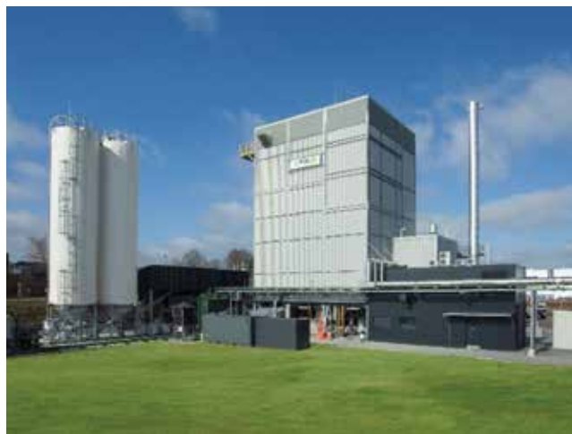
▲ Figure 2. This biomass pyrolysis plant uses the plant-in-a-box building concept, as the building's external walls are directly integrated with the modular skid structure.
