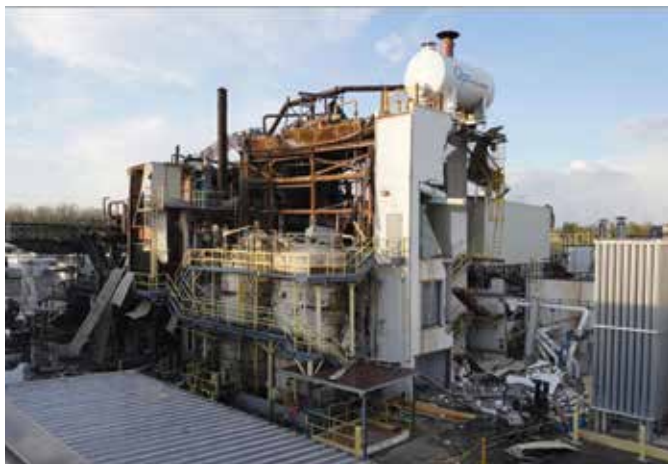
▲ An explosion and fire devastated a resin facility in Columbus, OH. Read U.S. Chemical Safety and Hazard Investigation (CSB) report No. 2021-04-I-OH for more information.
