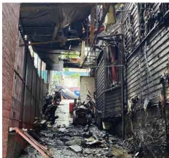
▲ This is the aftermath of a fire started by lithium-ion batteries. Image courtesy of the New York City Fire Dept.
