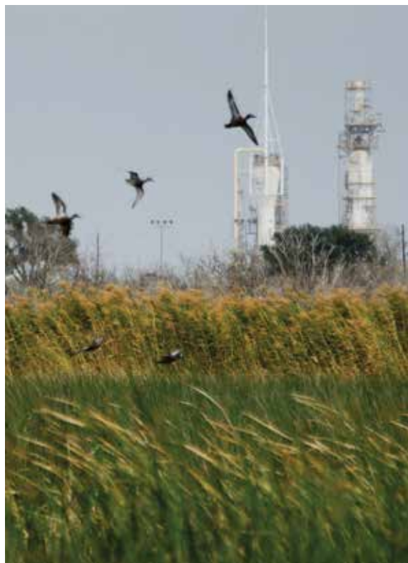
▲ Figure 1. The constructed wetlands within the buffer zone area of an operating facility were used to meet requirements for wastewater treatment instead of a more traditional sequencing batch reactor.
