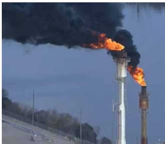
▲ Figure 1. Flaring is one of the most visible forms of waste at a refinery. In this photo, a refinery power outage has resulted in a flaring event with smoke visible for miles.
