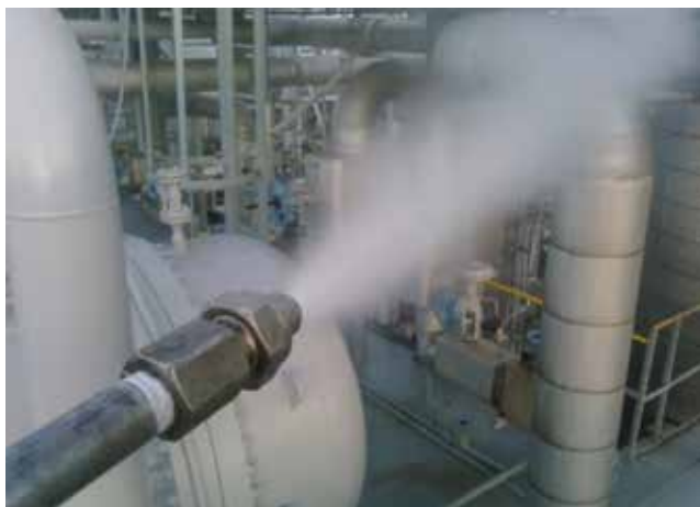
▲ Figure 9. Use an aerosolizing spray quill for liquids in slipstreams.
