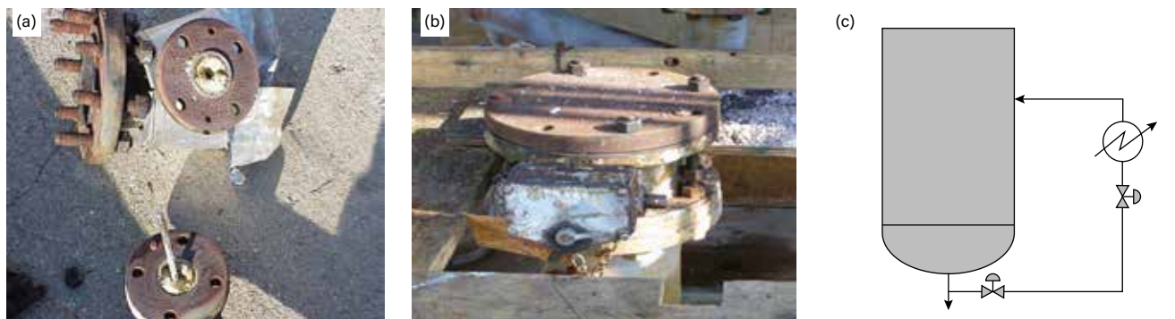
▲ Figure 4. Some examples of low-flow areas include (a) a level bridge, (b) a relief valve standpipe, and (c) a valved-off reboiler.
