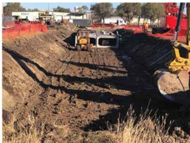
▲ **Figure 3.** Alluvial clays were encountered during installation of a new storm drain in Salina, KS. This site is located on a former Air Force base where metal-cleaning solvents were released from cleaning of aircraft on the tarmac, cleaning of parts in buildings, and landfills. The site has been investigated for potential impacts to indoor air and municipal groundwater. Photo courtesy of Tim Rogers.
