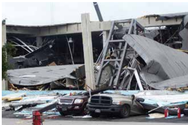
▲ A natural gas explosion at a meat processing plant caused a structural collapse and an ammonia release. Image courtesy of the U.S. Chemical Safety and Hazard Investigation Board.
