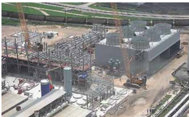
▲ Figure 3. The Petra Nova carbon capture and sequestration project is designed to capture approximately 90% of the CO 2 from a 240-MW slipstream of fluegas and use or sequester approximately 1.4 million m.t. of greenhouse gas per year. Image and data courtesy of the U.S. Dept. of Energy (DOE).
