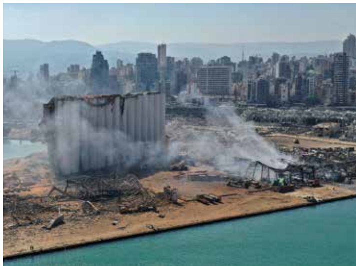
▲ After sitting in a warehouse for more than six years, a stockpile of ammonium nitrate (AN) exploded and caused severe damages in Beirut, Lebanon.
