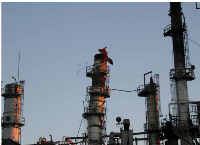
▲ Mononitrotoluene (MNT) exploded in this vacuum distillation tower while it was shut down. Image courtesy of the U.S. Chemical Safety and Hazard Investigation Board (CSB).
