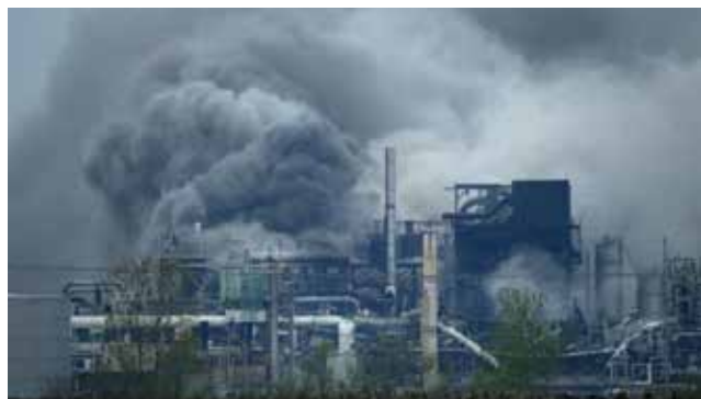
▲ Figure 3. Human error was a major factor in the release of highly flammable vinyl chloride that caused an explosion at a polyvinyl chloride (PVC) production unit. Source: (10).
