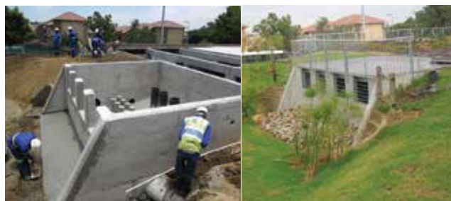
▲ Figure 4. Tupelovox Pty. Ltd. constructed a rainwater harvesting and treatment system capable of capturing 12 million L/yr of stormwater. These photos show the stormwater sediment trap during and after construction. Photos courtesy of Eugene Sihle Ngcobo.
