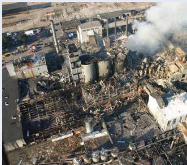
▲ Poor housekeeping at this Port Wentworth, GA, sugar mill exacerbated an incident that killed 14, injured 38, and destroyed the plant.
