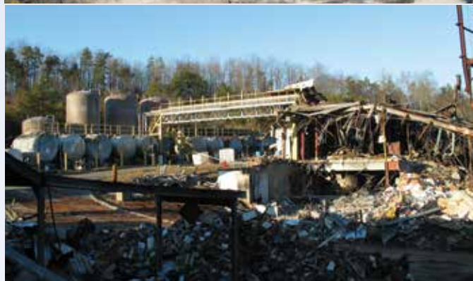
▲ Runaway reactions at other process facilities in Jacksonville, FL (top), and Morganton, NC (bottom), also caused extensive damage.
