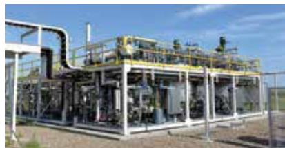
▲ The new processing facility at Iowa State Univ.'s BioCentury Research Farm for production and commercialization of soybean and glycerin-based biopolymers has a production capacity of 500 gal/day.
