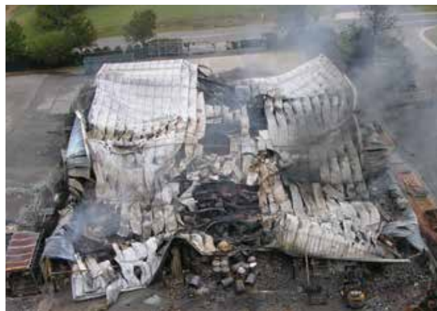
▲ Figure 6. The release at this TSDF destroyed the facility and forced residents nearby to evacuate.
