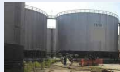
◀ Photo 1. A spark from hot work ignited vapors leaking from this spent sulfuric acid tank.
