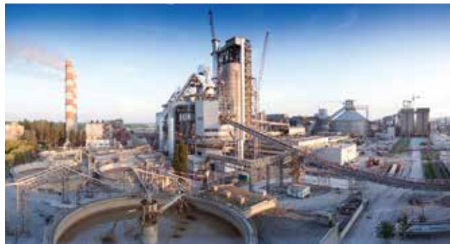
▲ Cement plants are large emitters of carbon dioxide that could use carbon mineralization to curb emissions.
