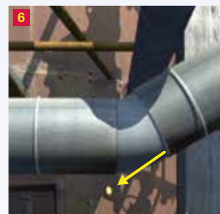
Drips from insulated pipe
