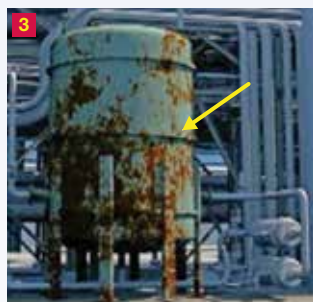
Rusting and corrosion of equipment
