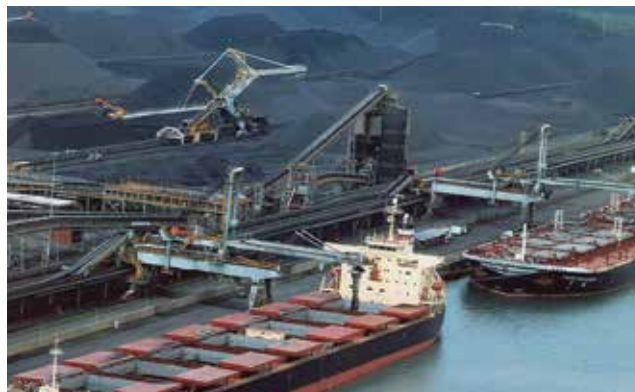
▲ Figure 5. The Richards Bay Coal Terminal, in KwaZulu-Natal Province on the Indian Ocean, is Africa’s largest coal exporting facility. Ninety-two percent of the coal consumed on the African continent is mined in South Africa. Photo courtesy of Richards Bay Coal Terminal.
