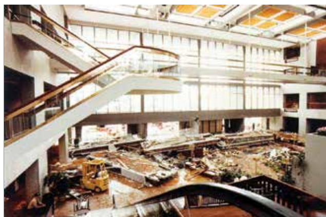
▲ Figure 1. Two suspended walkways in the Hyatt Regency Kansas City collapsed as dozens of party-goers dancing on them caused them to sway and vibrate — subjecting them to a larger-than-expected dynamic load. Source: MatDL: Failure Cases Wiki, http://matdl.org/failurecases/File%253AHyatt.3.jpg.html
