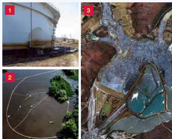
▲ (1) A damaged storage tank and a spill into a containment dike; (2) Spill containment and cleanup efforts; (3) Aerial view of the Kingston spill.
