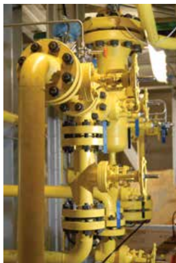
▲ Figure 4. Flanged joints are typically only available in large pipe sizes, and nearly impossible to find below 0.5 in. IPS. Photo courtesy of Zeton, Inc.
