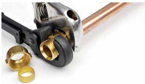
▲ Figure 16. Use a holdback (black wrench) whenever tightening or loosening a fitting on threaded piping to avoid excess stress on adjacent fittings.
