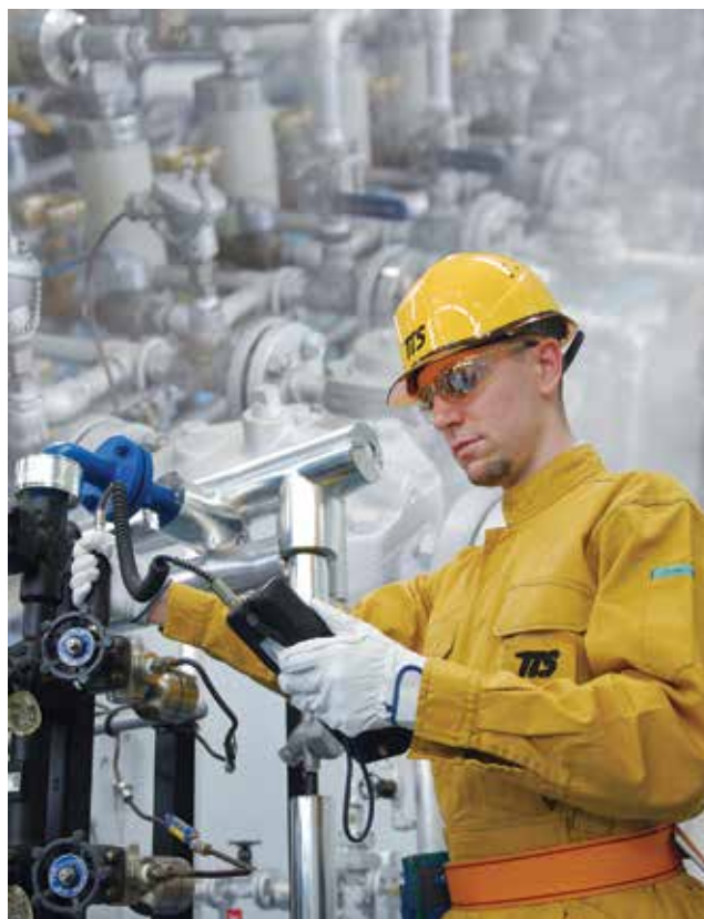
▲ Figure 1. The steam-trap survey is the key component of a steam-trap management program. However, a plant should not jump into performing the survey without proper planning and preparation.
