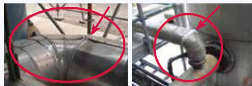
▲ Examples of damaged insulation
