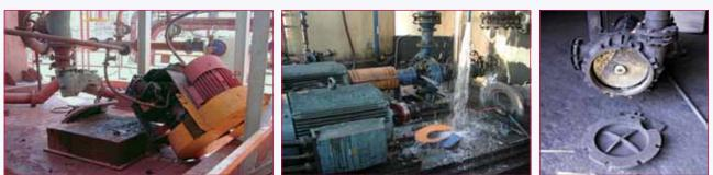
The answer must be yes, or we would not have a Beacon on this subject. The centrifugal pumps in the pictures are all water pumps that exploded. The explosions did not occur because of any contamination or chemical reaction with something that was not supposed to be in the pump. In fact, explosions like this have happened with very pure water in boiler feedwater pumps, condensate pumps, and deionized water pumps.
