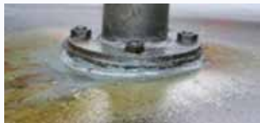
▲ Is something leaking from this flange?
