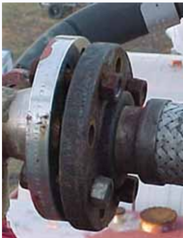
▲ Bolts missing from a flange.
