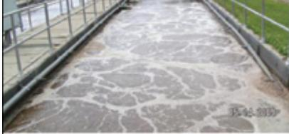
Pulsair Chemical and Wastewater Mixing Systems efficiently mix aeration tanks, anoxic basins, sludge tanks, and chemical tanks using up to **75% Less Energy** than conventional mechanical mixers...and there are no immersed impellers, shafts, gears, seals or any other moving parts in the tank.
