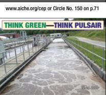
Pulsair Chemical and Wastewater Mixing Systems efficiently mix aeration tanks, anoxic basins, sludge tanks, and chemical tanks using up to 75% Less Energy than conventional mechanical mixers...and there are no immersed impellors, shafts, gears, seals or any other moving parts in the tank.
